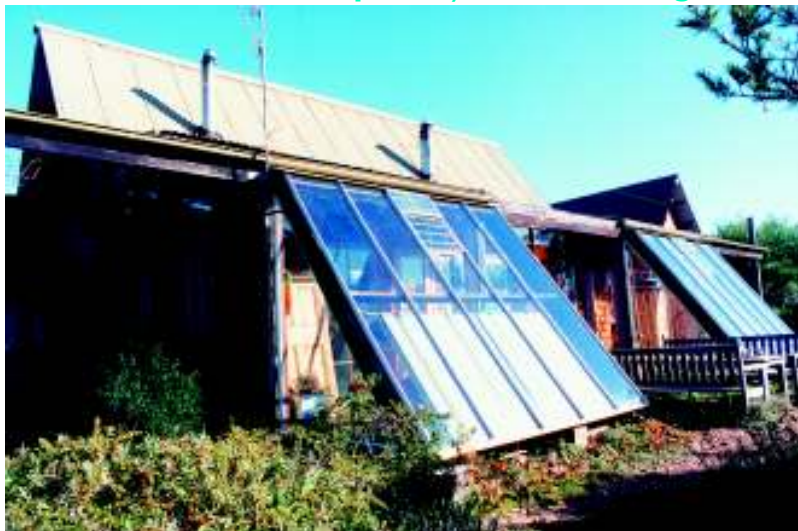
Cold climate solution — glasshouses face sunward on this mudbrick and timber house to warm the interior in winter. Heat is vented off in summer. A cosy sitting and dining nook was placed between glasshouses.
